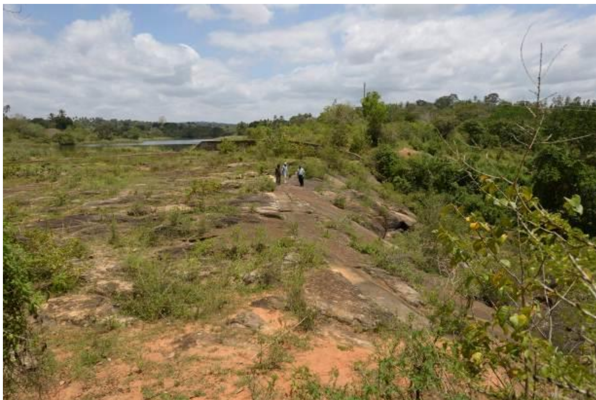
The spillway, the local Sandstone and drop in the riverbed
