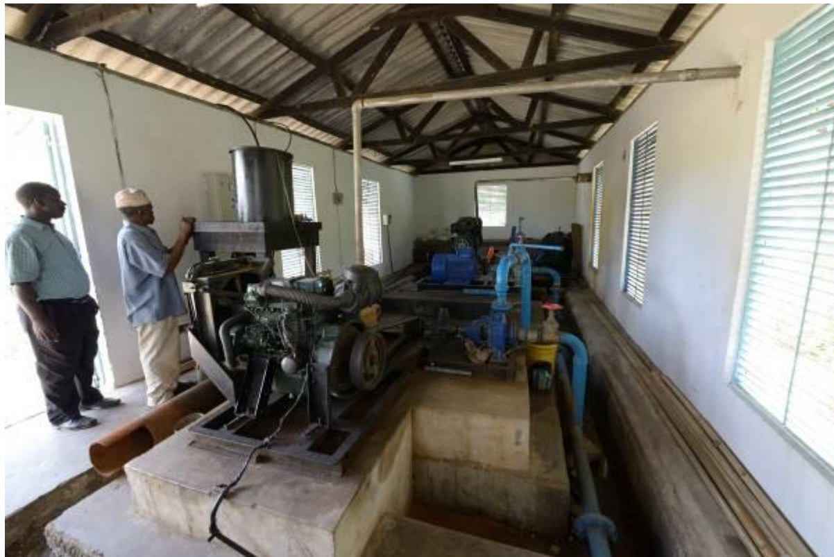
Photo sheet 13 – The Intake and pumping house
