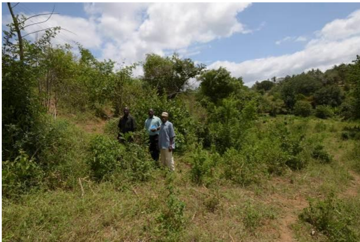
The external slope of the dam
